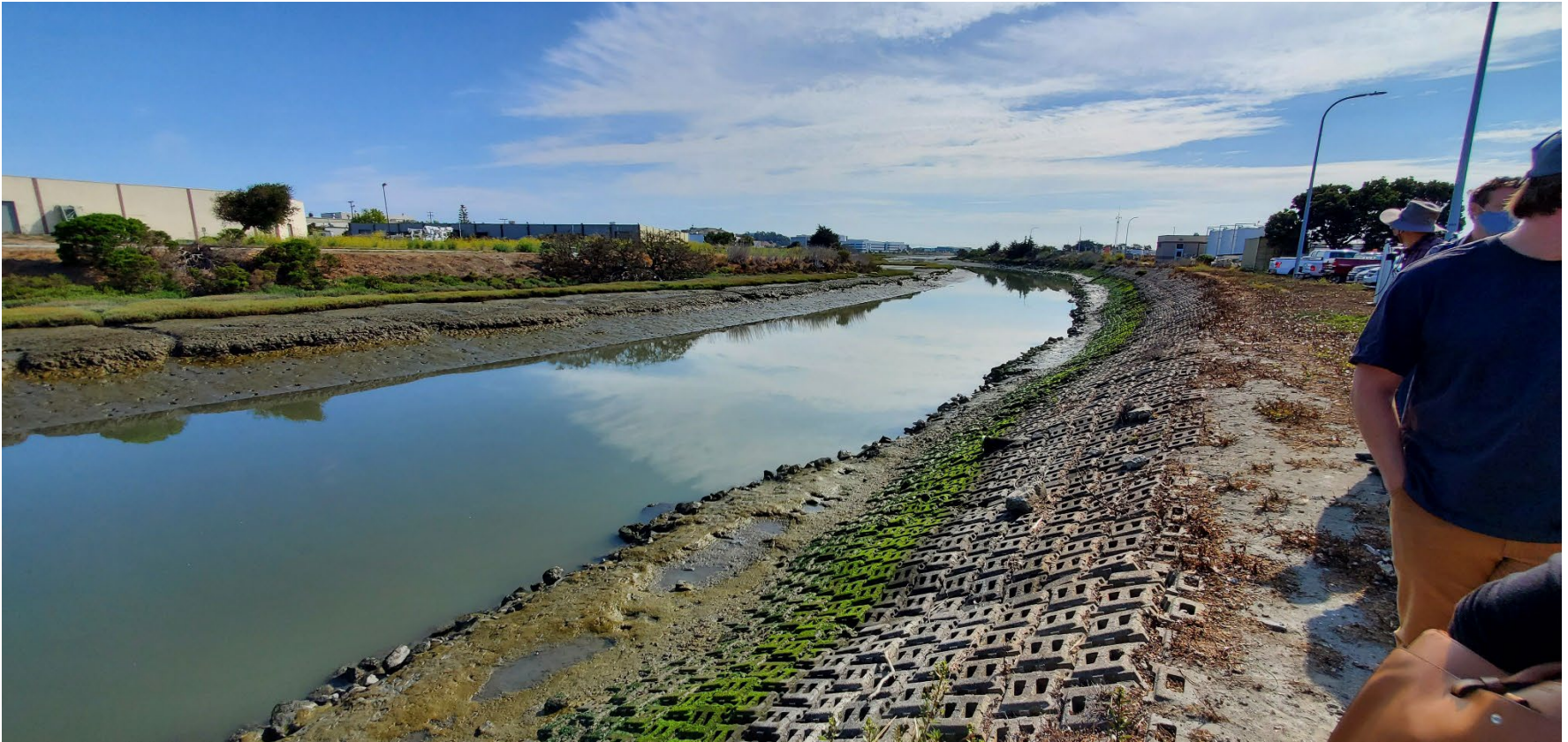
A1. View of Colma creek channel looking downstream from the south (WQCP) side.
