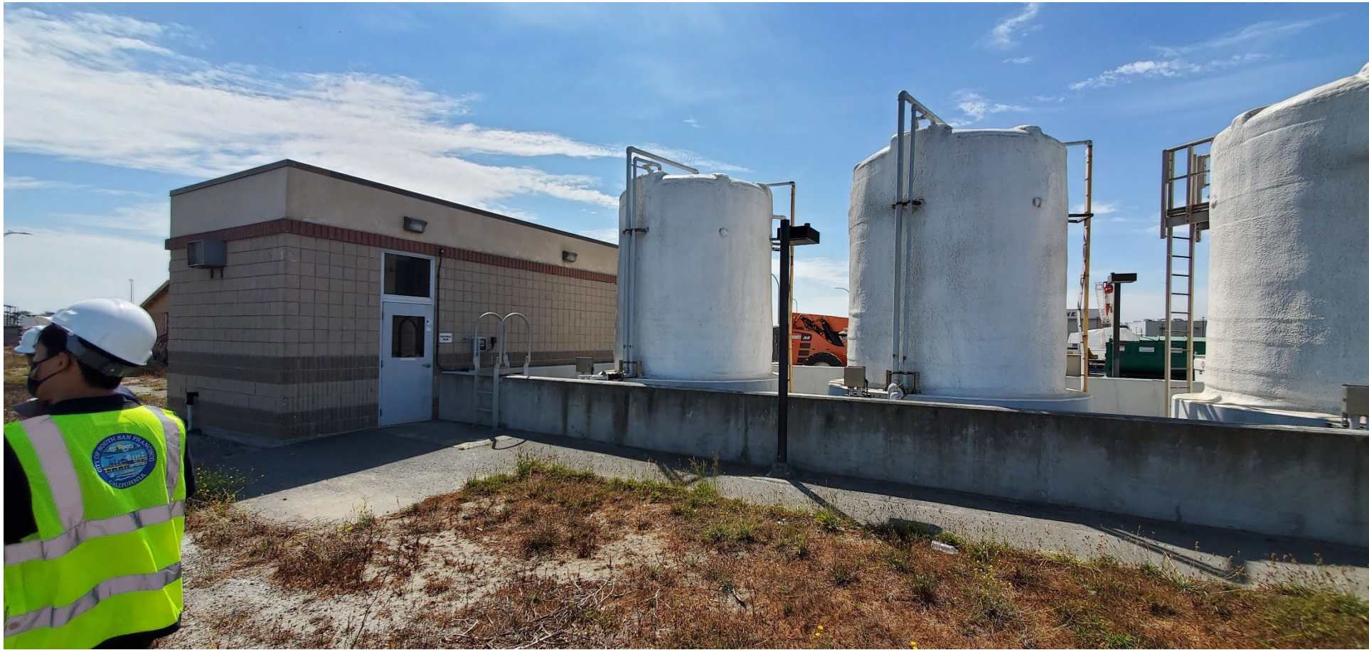
A4. Some facilities have a short wall to keep water out.
