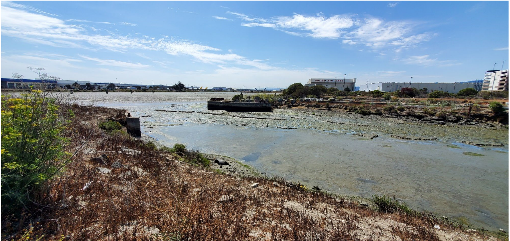
A5. View looking into the piers on the south side of the WQCP area.
